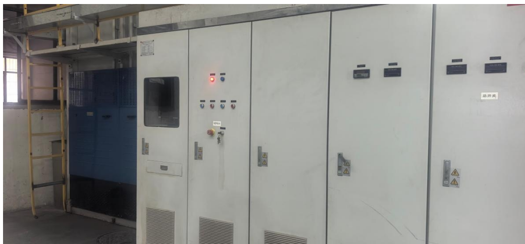
Fig.9 Heat soak oven temperature control machine
